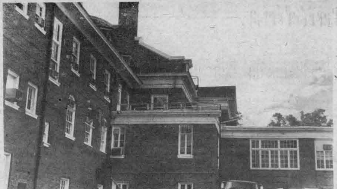
NORTHERN EXPOSURE: The Old Administration building has stood as an architectural landmark since 1910. Present attempts are being made to preserve it as an historical landmark [Photo by Rich Shumacher].
